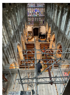
View from the top of the scaffolding
