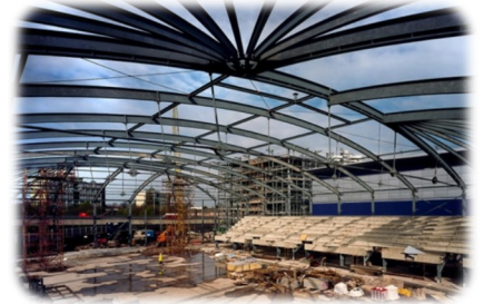
The start of the Coventry Sports Stadium.
